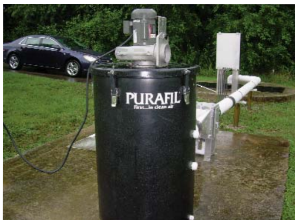
PURAFIL® DRUM SCRUBBER (DS) 300 REMOVED THE BAD ODORS RELEASED BY THE WET WELL
